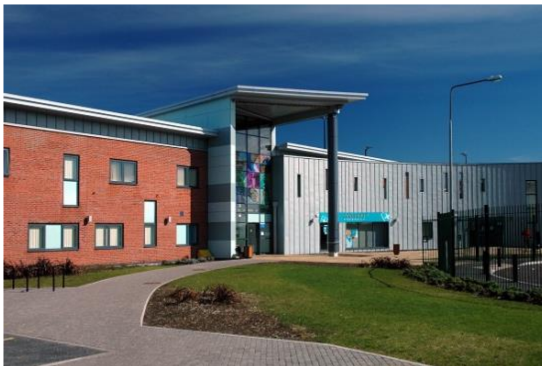
Figure 2: Dr Maassarani & Partners - Tower Hill main site
